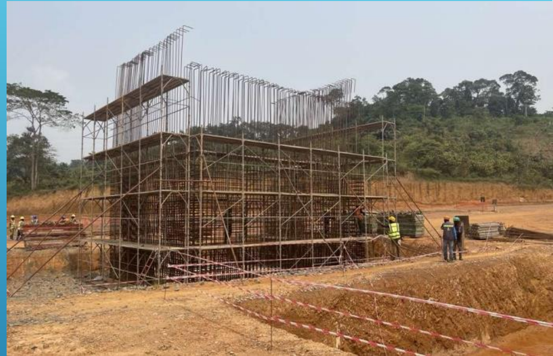
Road overbridge construction near Amantin
