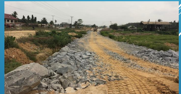
Soil stabilization near Aboso
