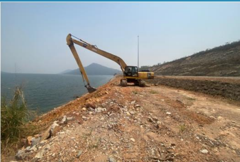
Mpakadan Railhead (Km 97+000) – Slope dressing
