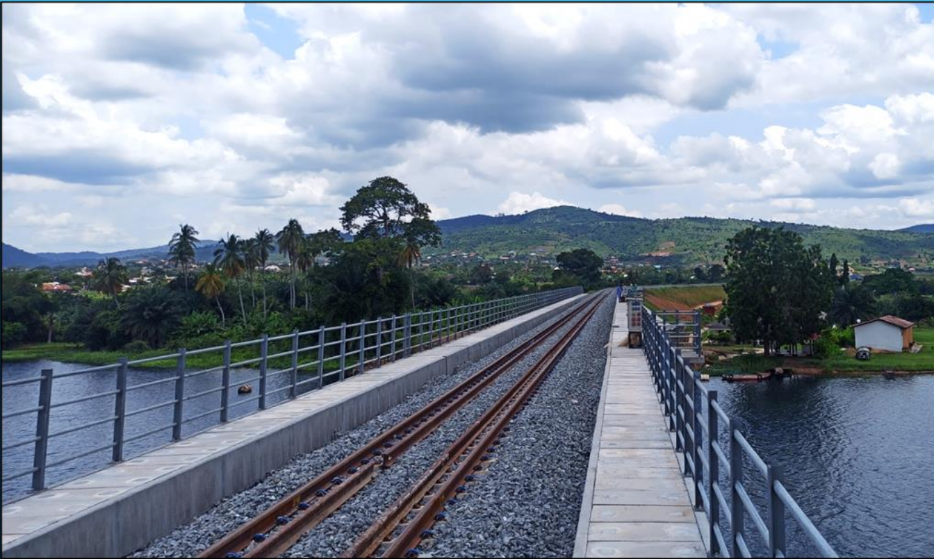
Handrails fixed and tracks laid
