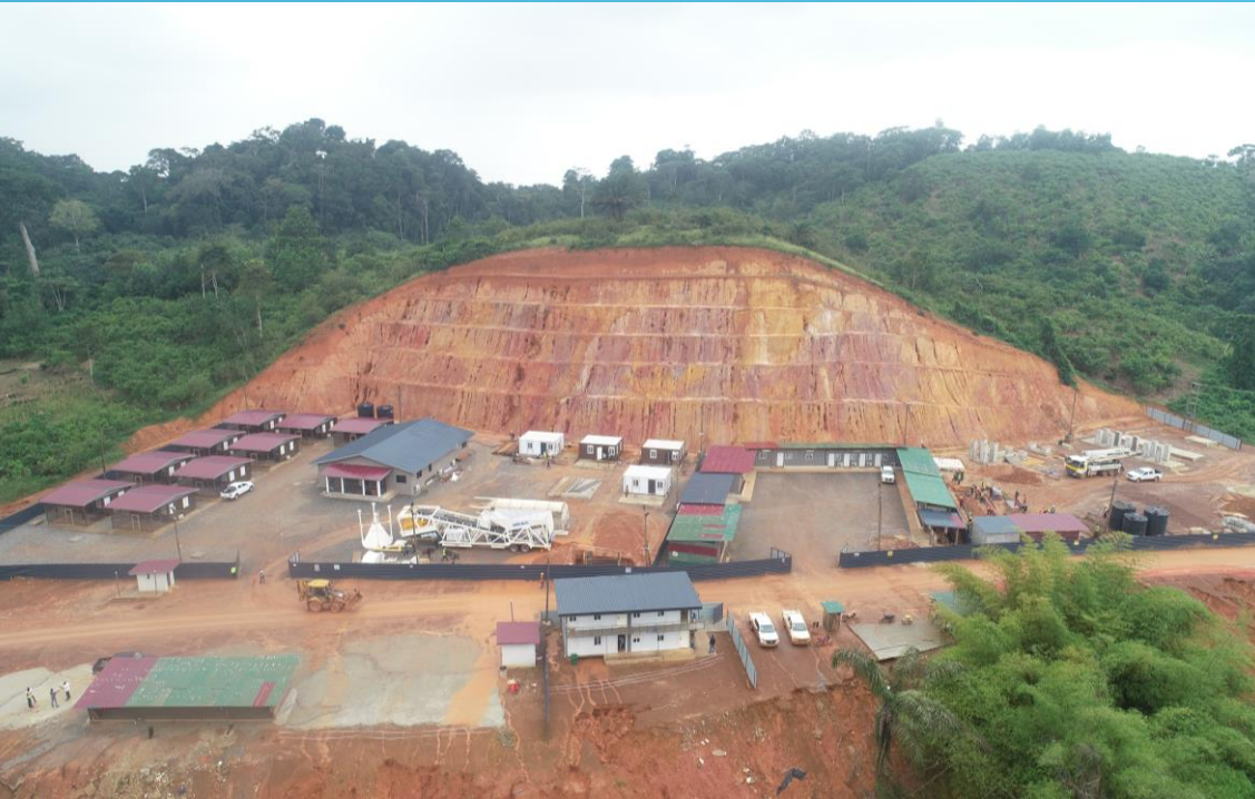
Contractor site office in Benso
