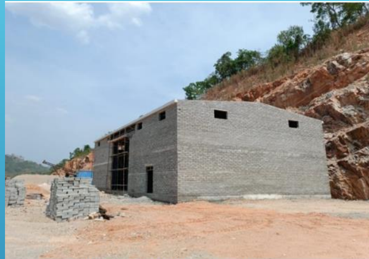
Mpakadan Railhead (Km 97+000) – Warehouse
