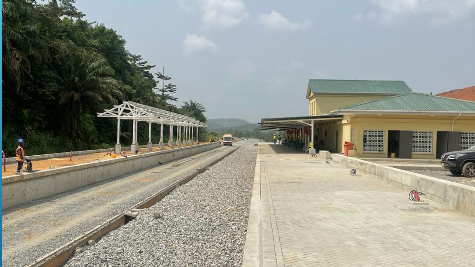
Manso Railway Station: 98% complete
