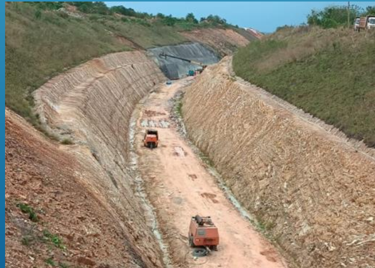
Cut section (Km 94+200 – Km 94+600 approx.) – Overview
