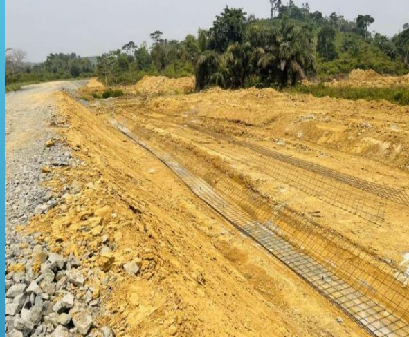
Drains being reinforced
