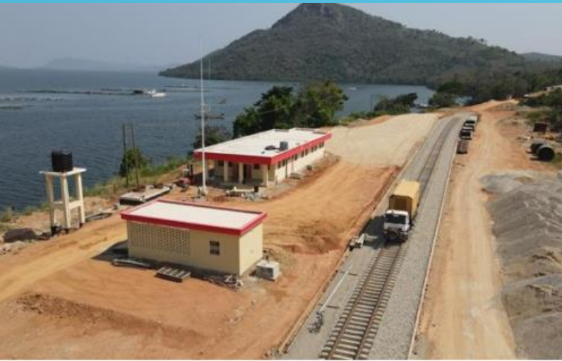
Mpakadan Railhead (Km 96+000) – Operational Building
