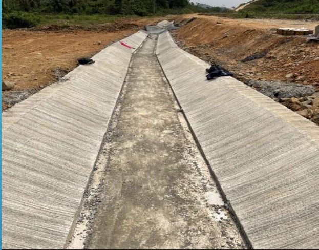
Trapezoidal drain construction
