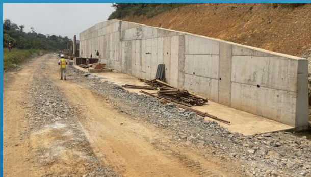
Retaining wall construction near Amantin
