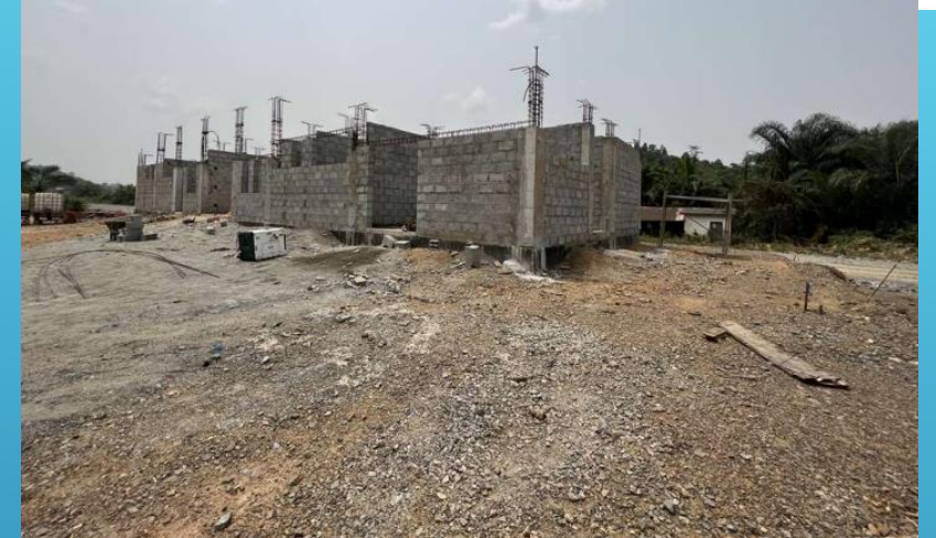
Amantin Station under construction
